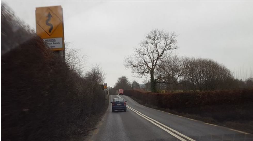
Figure 1-11 N13 North of Stranorlar with no footway or Hardstrip
