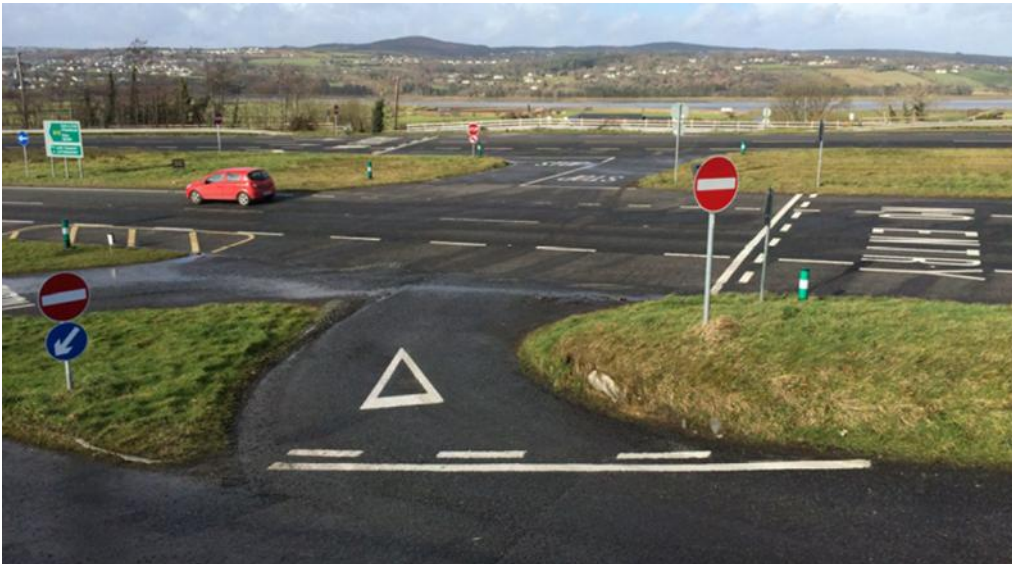
Figure 2.18: Trimragh Junction on the N13 Dual Carriageway
