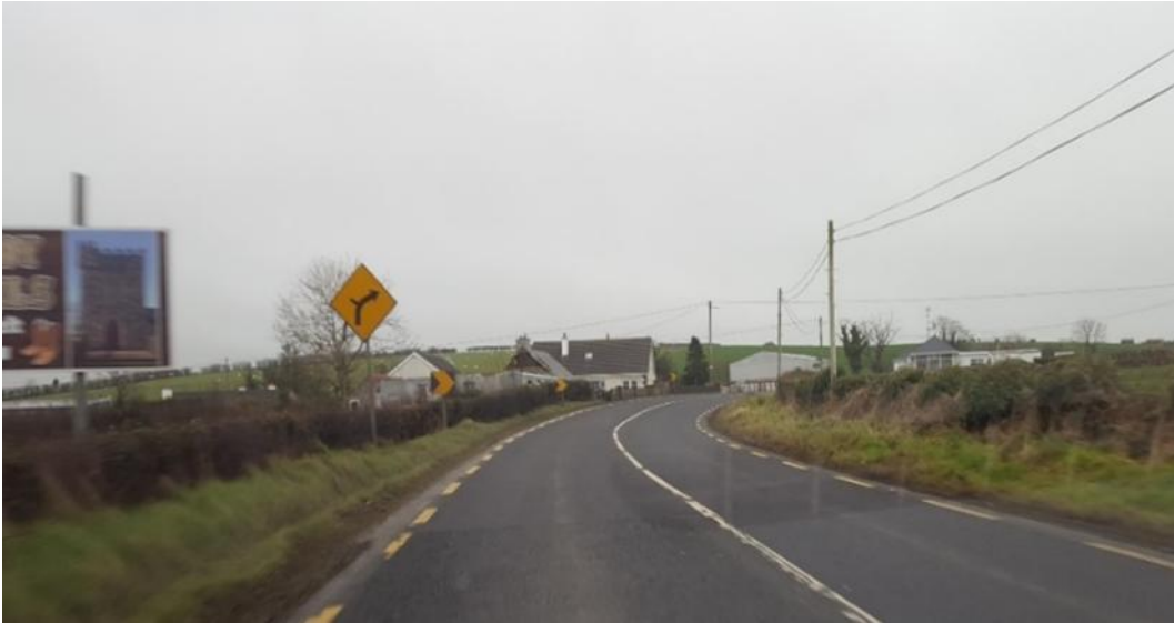
Figure 2.19: N14 between Manorcunningham and the R236
