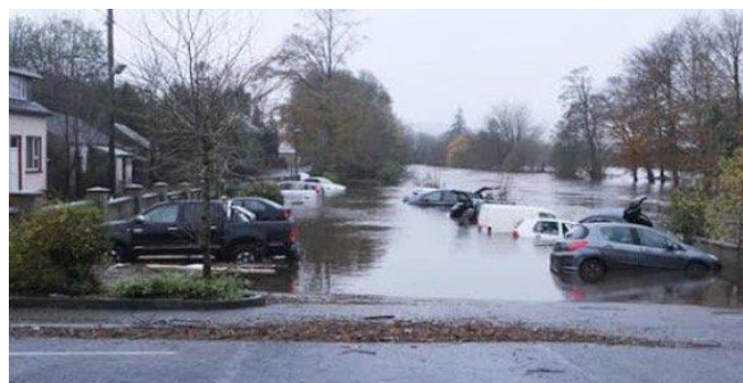
Image 3.4 Flooding at Jackson's Hotel, Ballybofey (downstream of proposed crossing)
