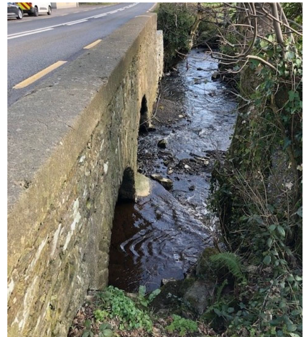
Photo 4: Downstream of existing N15 Culvert
