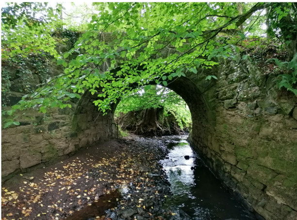
Photo 5: Upstream of existing Railway Culvert
