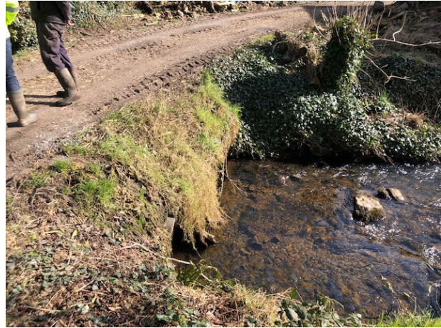
Photo 2: Downstream of existing Pipe Culvert
