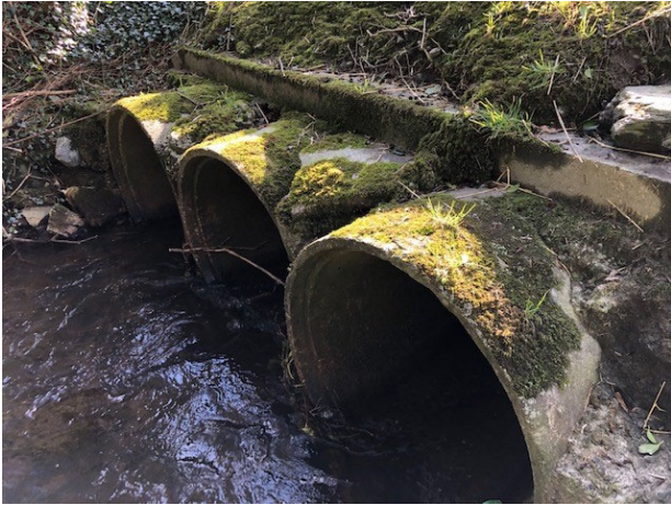
Photo 1: Upstream of existing Pipe Culvert
