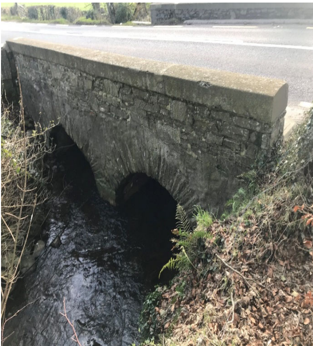
Photo 3: Upstream of existing N15 Culvert
