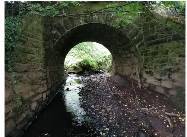
Photo 6: Downstream of existing Railway Culvert
