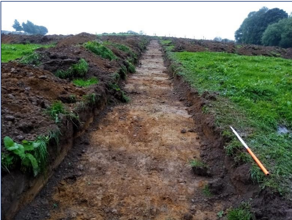
Plate 4: Example of a machine dug trench (T1); facing south-southwest
