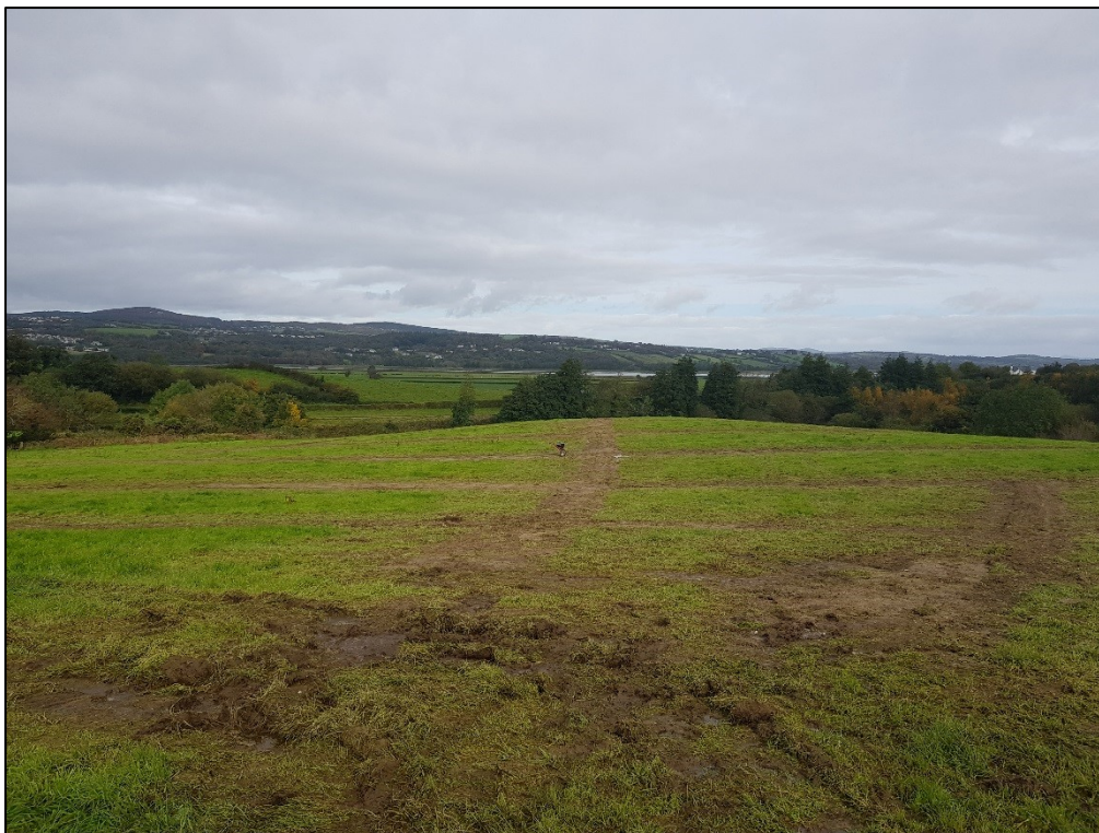
Plate 5: Backfilling completed at Trimragh with re-seeding in progress; facing north
