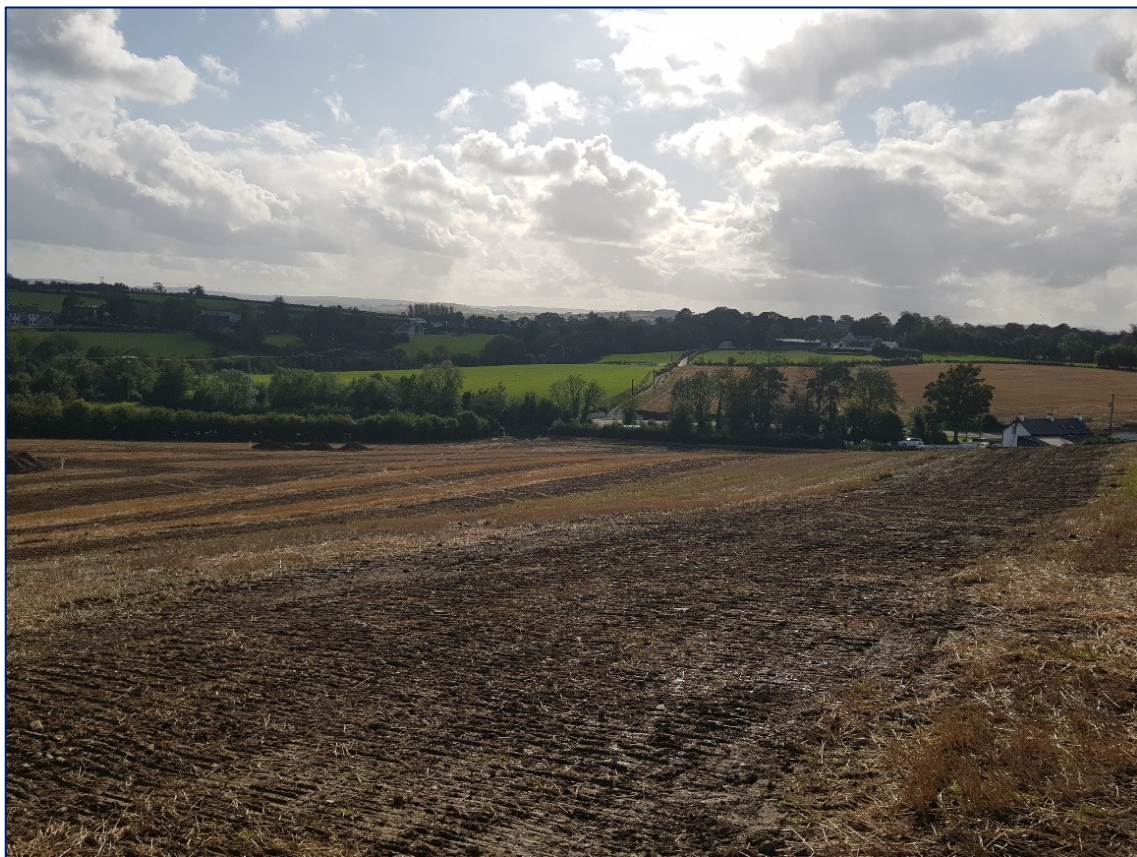
Plate 12: Backfilling nearing completion at Carnshannagh; facing west
