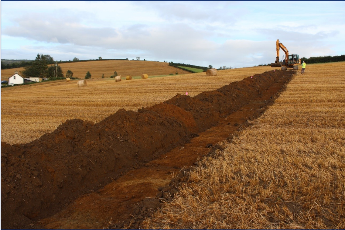
Plate 1: Example of trenching in the southern field (T37); facing northwest
