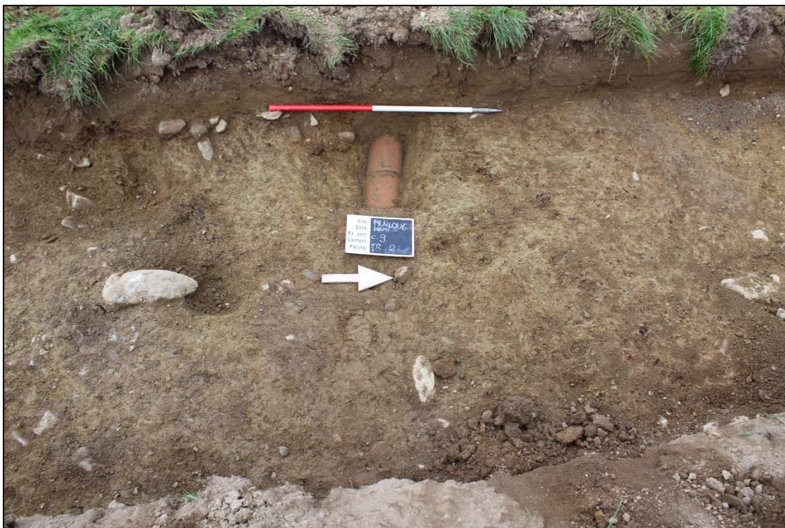
Plate 10: Modern drainage pipe C.9 (T21); facing west
