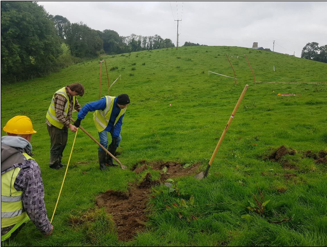
Plate 1: Commencing hand excavation of trenches (T24 and T25) under overhead powerlines
