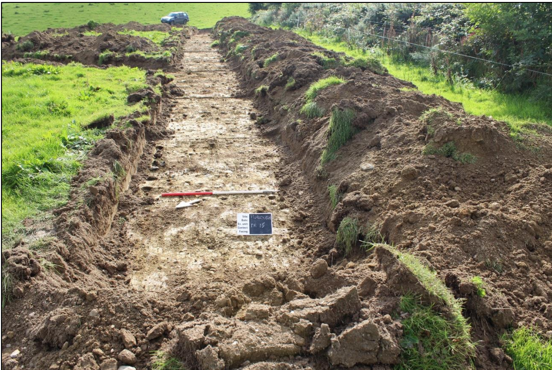
Plate 4: Example of machine-dug trench (T15); facing southwest
