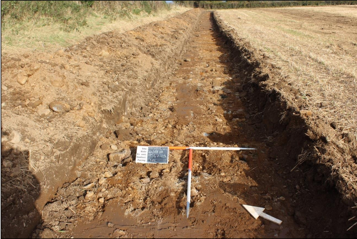
Plate 1: Example of trenching in the western field (T47); facing east
