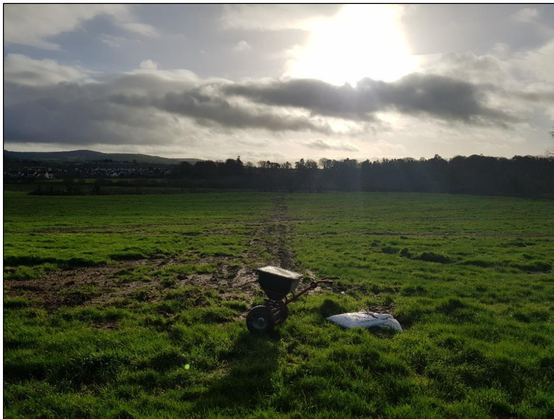
Plate 15: Backfilling complete at Curraghallane, with re-seeding in progress; facing south
