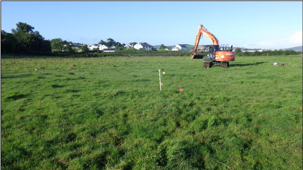
Plate 1: Pre-excitation view of test excavation area TA6, looking southwest.
