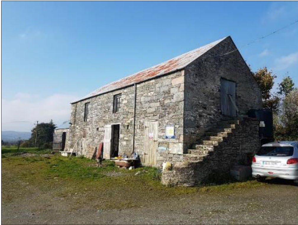
Plate S1-31: View of front elevation to outbuilding S1-BH02, Ch. 4+400, Drumboe Upper
