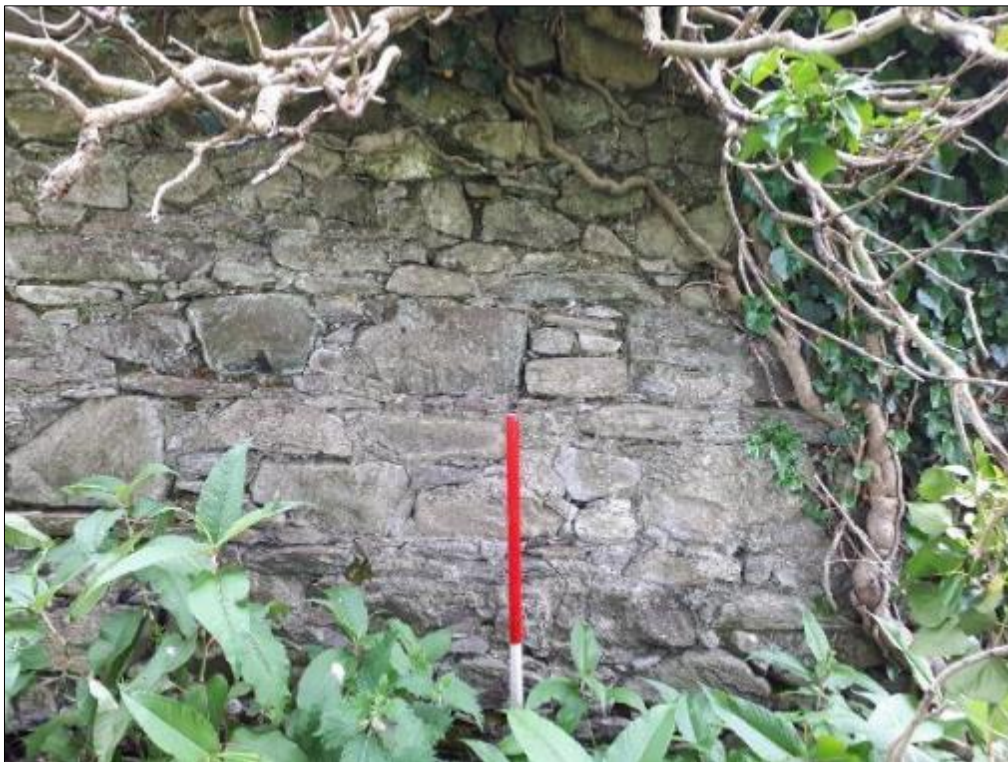
Plate S1-23: View of a putlog hole to northern wall of avenue, F-1-13, Drumboe Lower, Ch. 3+300
