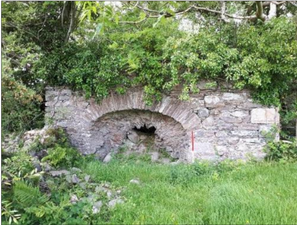
Plate S1-52: View of ruined lime kiln F-1-21 at Castlebane, west of Ch. 00 Side Rd (Mullandrait Link Rd)
