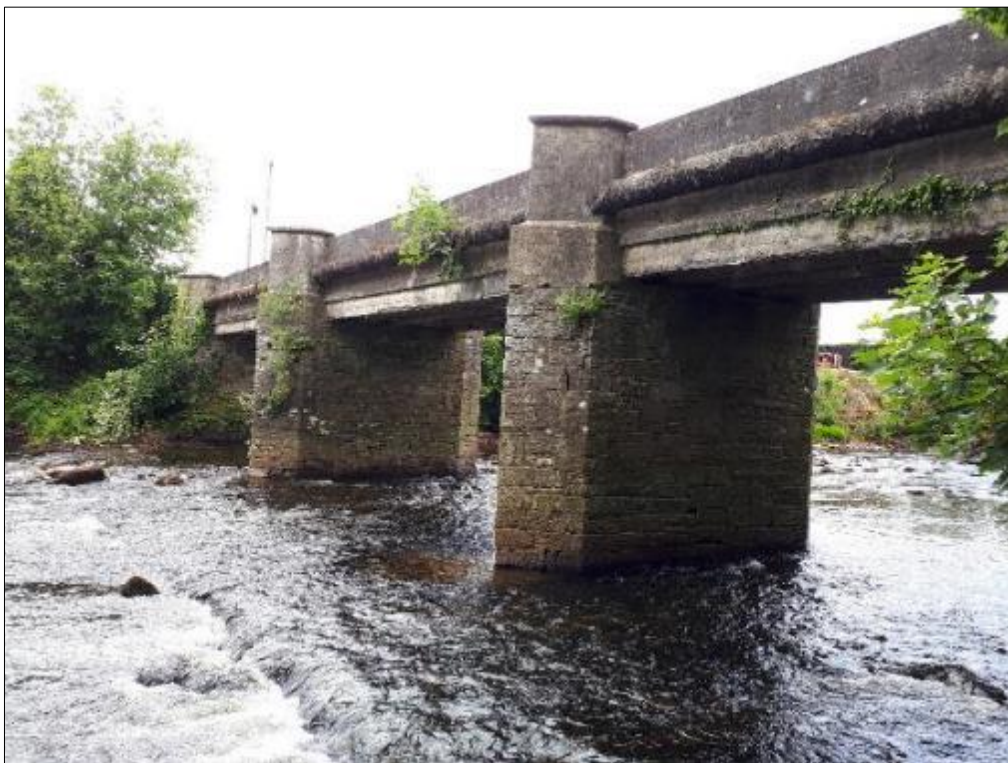
Plate S1-13: View of bridge from riparian area, facing south-southwest
