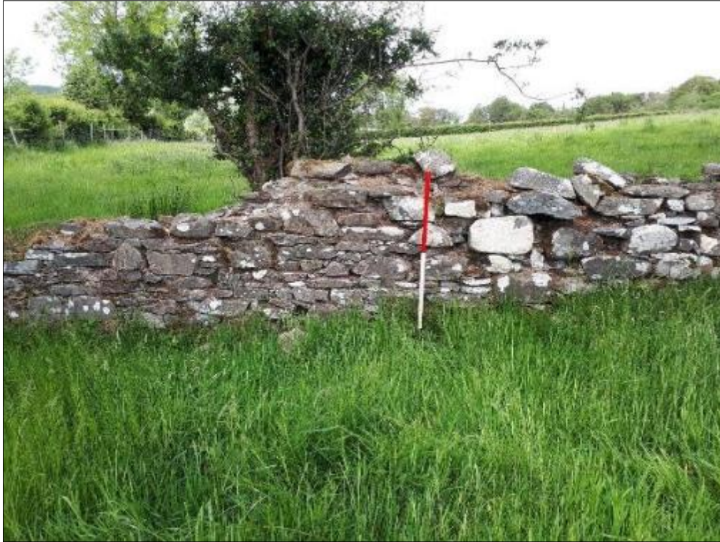
Plate S1-18: View of mortared wall F-1-11 at Ch. 3 +150, facing north
