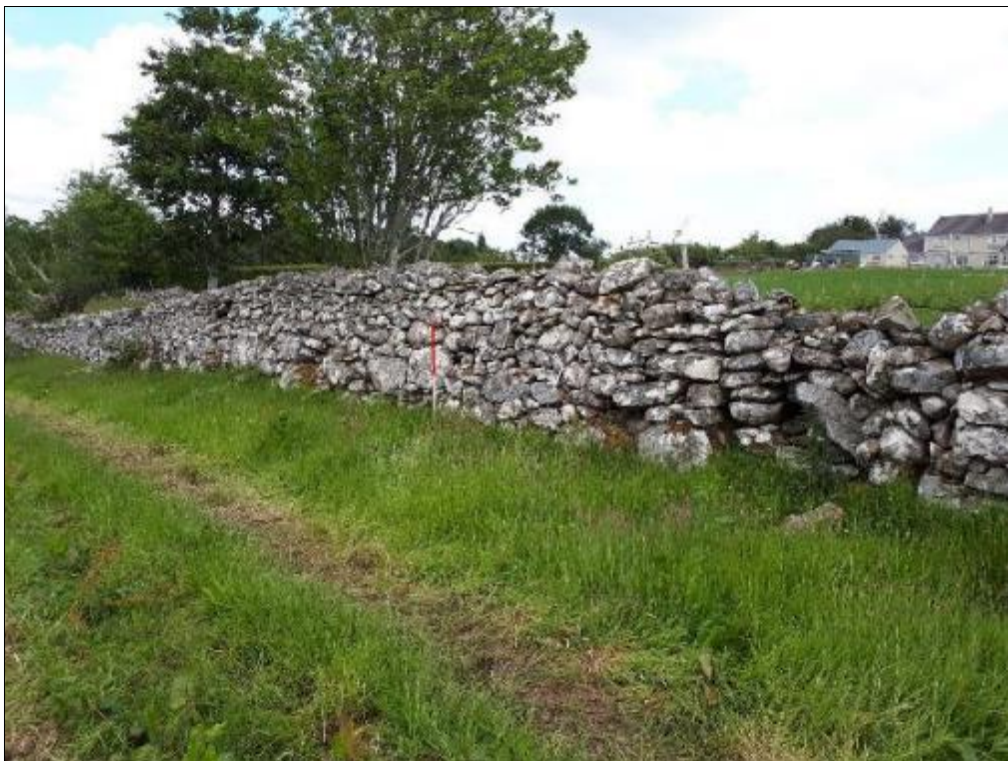
Plate S1-26: View of eastern stone wall field boundary (F-1-16) of the 'abbey field', facing northeast
