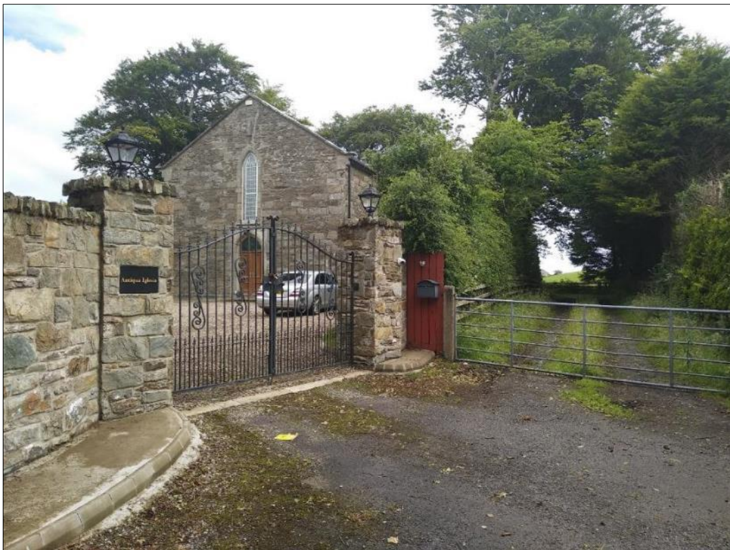
Plate S2-12: View of former COI church (NIAH 40905301) facing northeast
