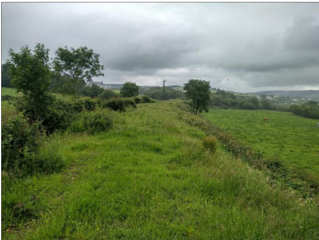
Plate S2-17: View of former Strabane to Letterkenny narrow gauge railway line (S2-BH04)
