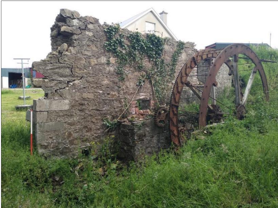
Plate S2-34: View of remaining wall elevation of mill structure NIAH 40905390
