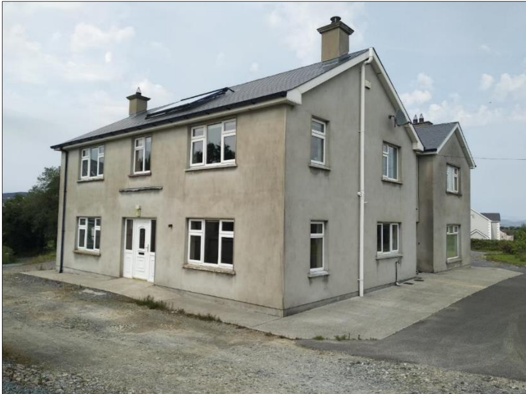
Plate S2-38: Side view of new houses at location of former NIAH recorded houses 40905339
