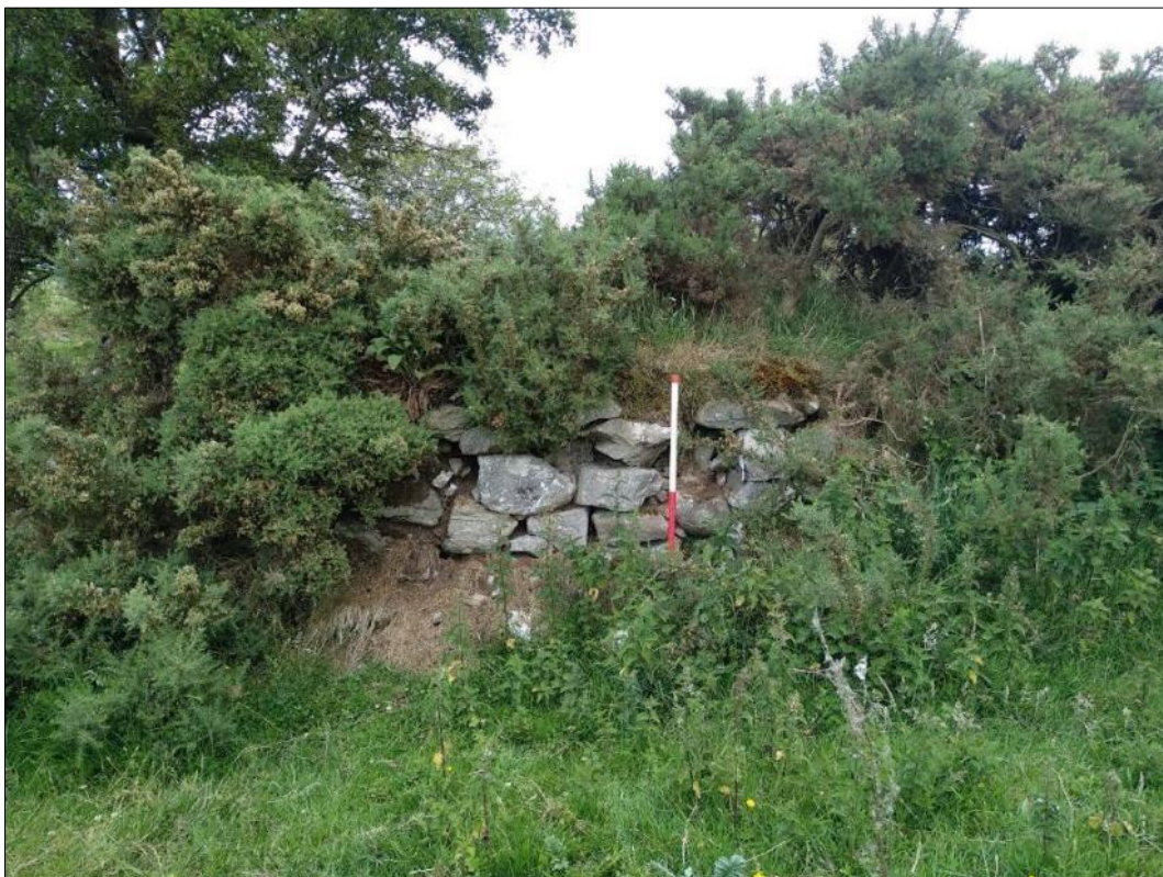
Plate S2-24: View of stone wall, (ITM approx. 618898, 911775) Ch. 0+300
