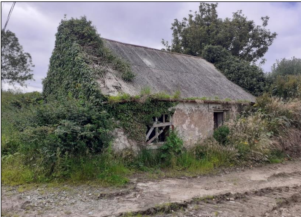
Plate S3-56: View to northwest of vernacular cottage at Ch. 9+400
