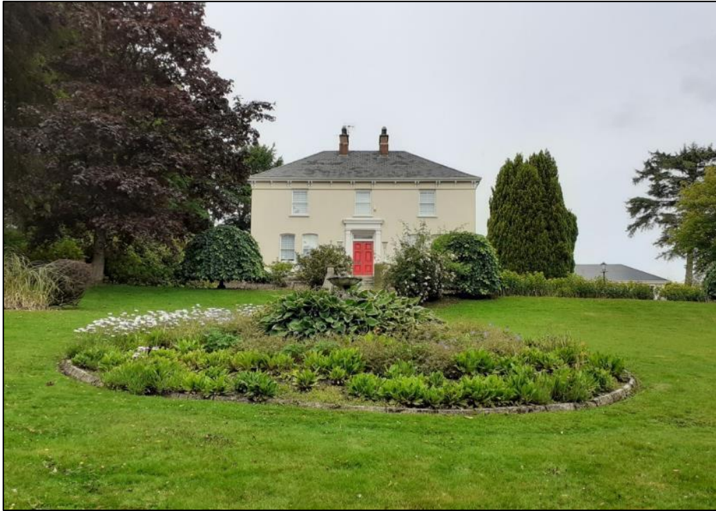
Plate S3-02: Front (east) elevation of Gort Presbyterian Manse (NIAH 40827011)
