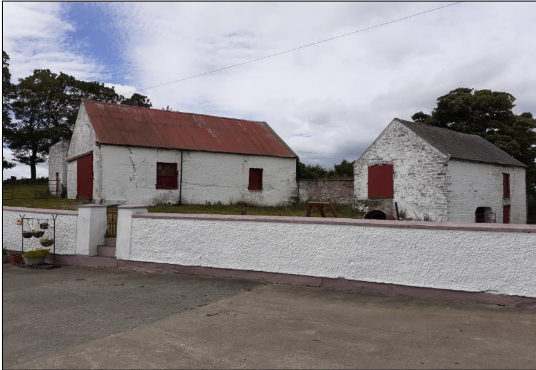
Plate S3-24: View to west of outbuilding (NIAH 40906245), northeast of Ch. 3+600
