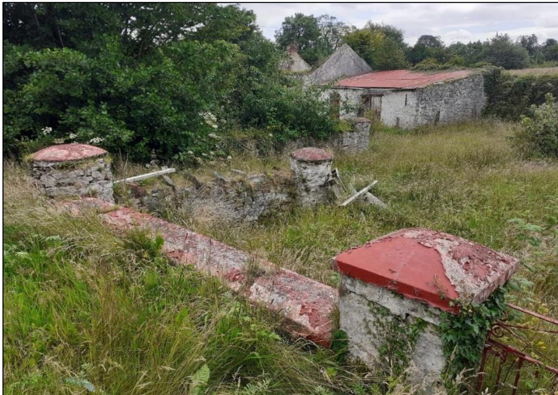
Plate S3-58: View to southwest of part of ruined vernacular complex along N14 (to northwest of cottage NIAH 40906262) southwest of Ch. 9+250
