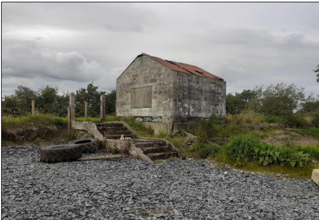
Plate S3-87: View to southwest of ancillary railway structure (NIAH 40834011) Ch. 14+100
