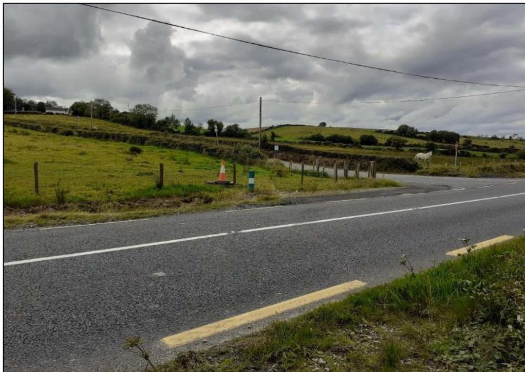
Plate S3-29: View to northwest, Ch. 4+200 – 4+500
