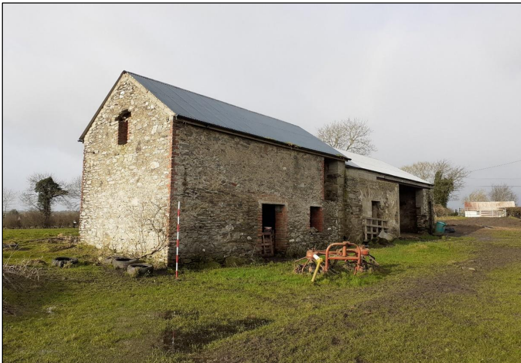
Plate S3-05 Vernacular stone outbuildings at 'Black Bush' Ref. M501
