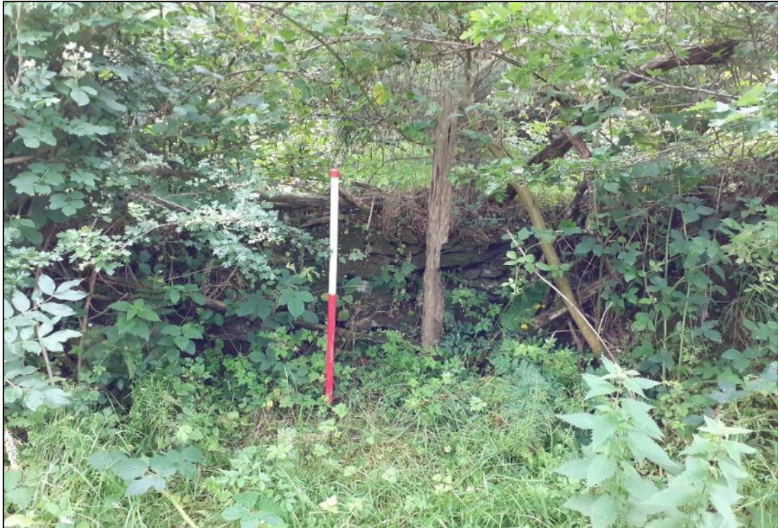
Plate S3-19: View to southeast of stone wall at Ch. 2+400
