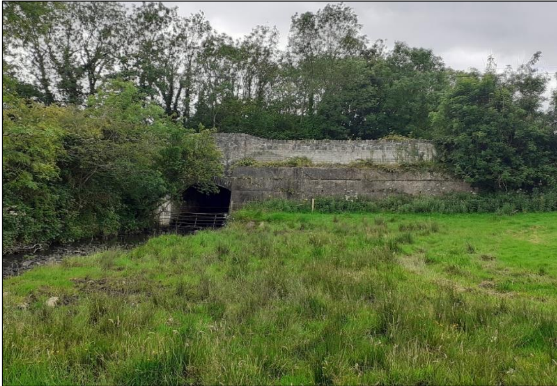
Plate S3-57: View to west of road bridge at Ch. 9+380
