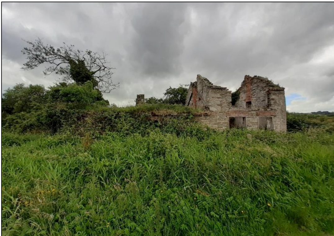
Plate S3-43: View to NW at Ch. 7+000 – 7+100 (F-3-09)
