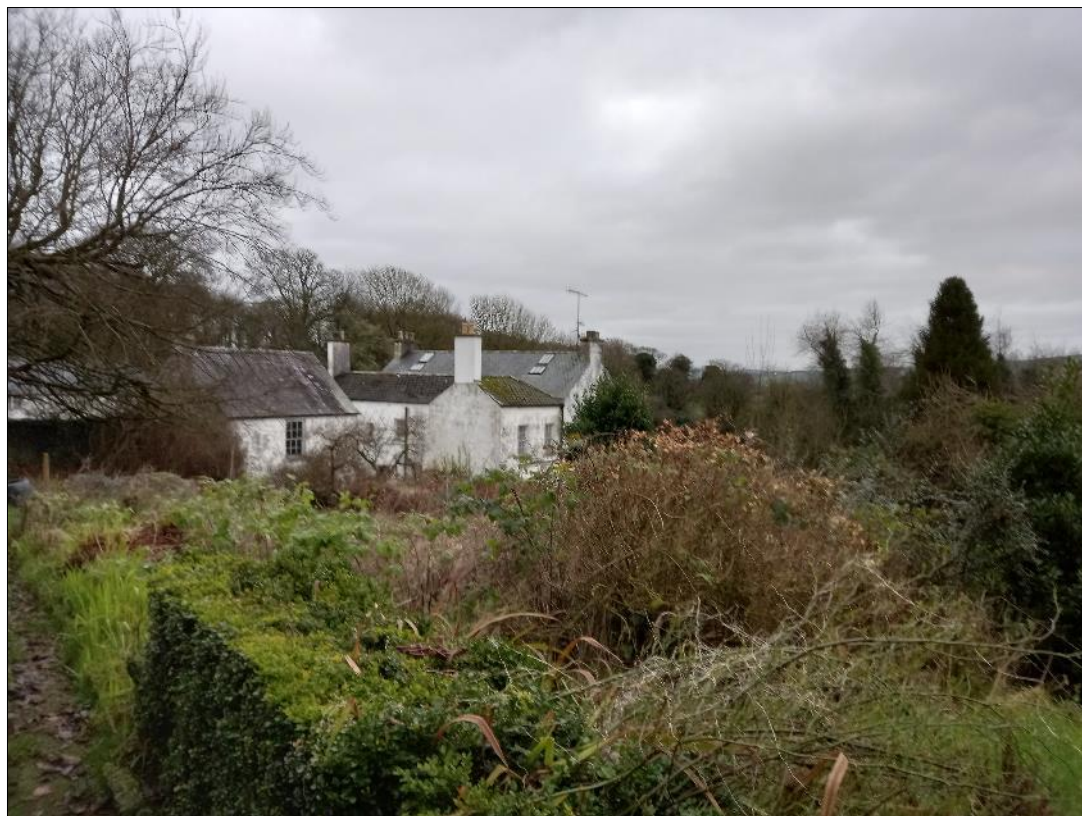
Plate S3-83: View to northeast across walled garden to rear of Cavanacor House and outbuildings
