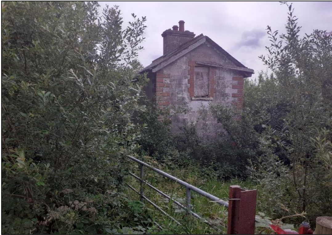
Plate S3-86: View to southeast of Station Masters House (NIAH 40834011) Ch. 14+100
