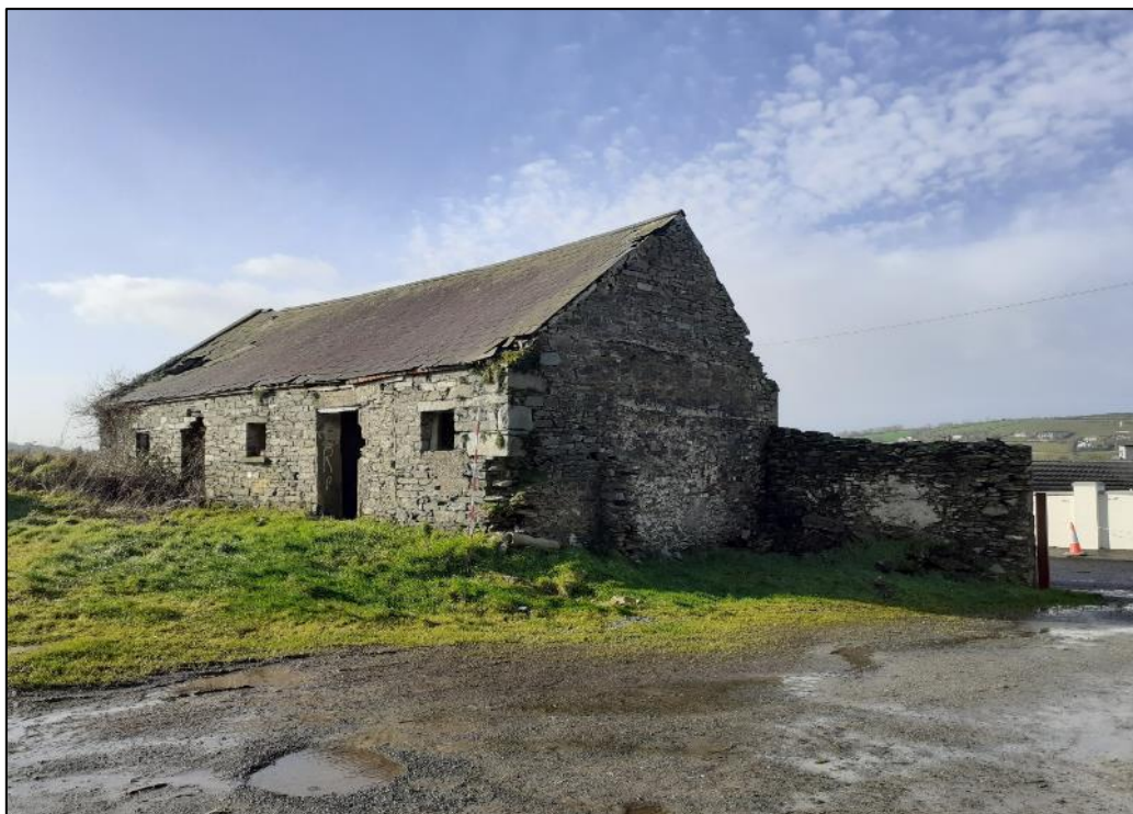
Plate S3-78: Vernacular stone outbuildings, M698 Tamnawood, facing southwest
