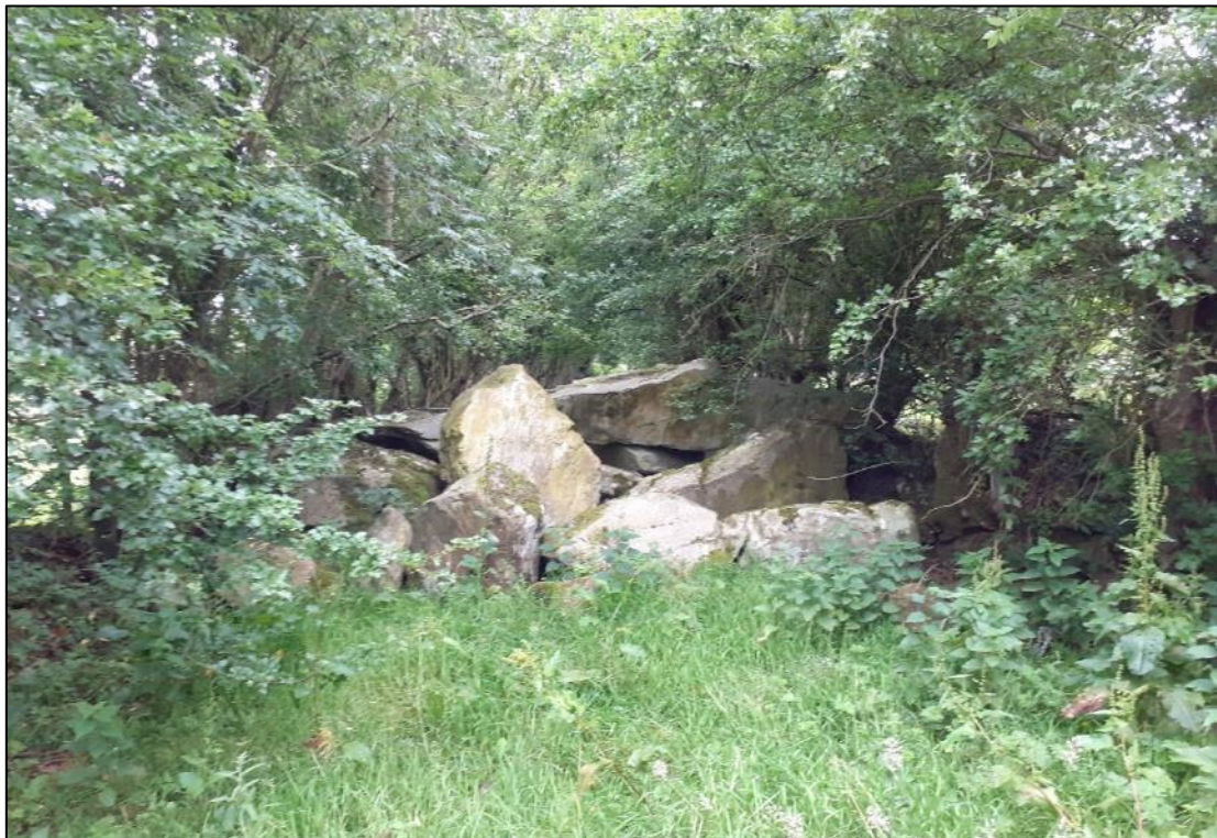
Plate S3-20: View to northeast of disused laneway blocked by large boulders Ch. 2+400
