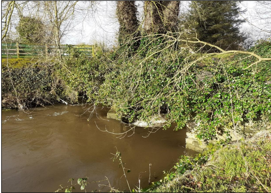
Plate S3-06 Connaghan's Bridge NIAH 40905456 (overgrown) facing southwest
