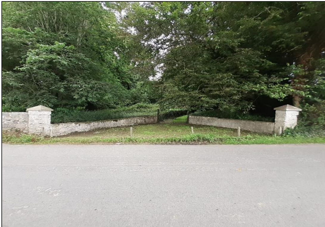
Plate S3-81: View to north of Cavanacor House west gate entrance
