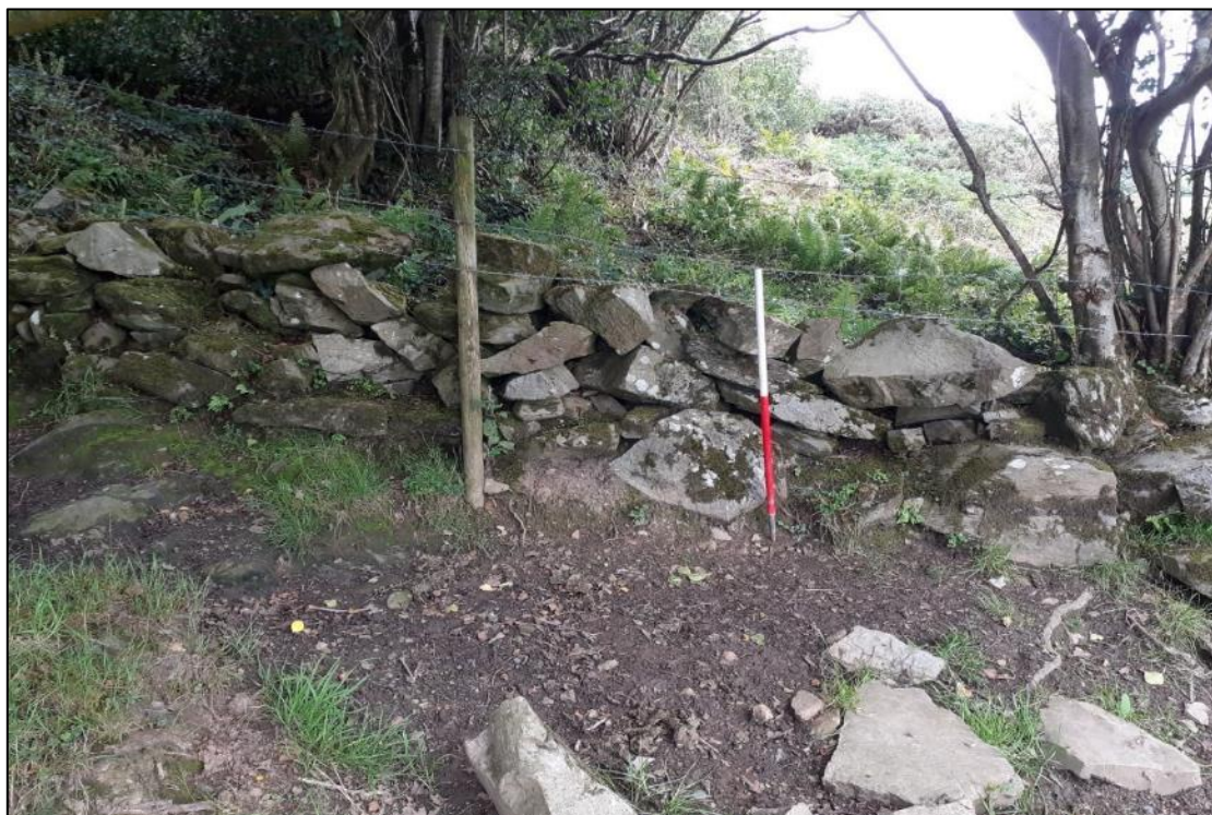
Plate S3-53: View to east of drystone wall at Ch. 8+800
