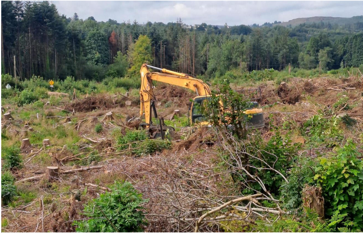
Apx Figure 16: Enhancement Works Taking Place at the time of Survey
