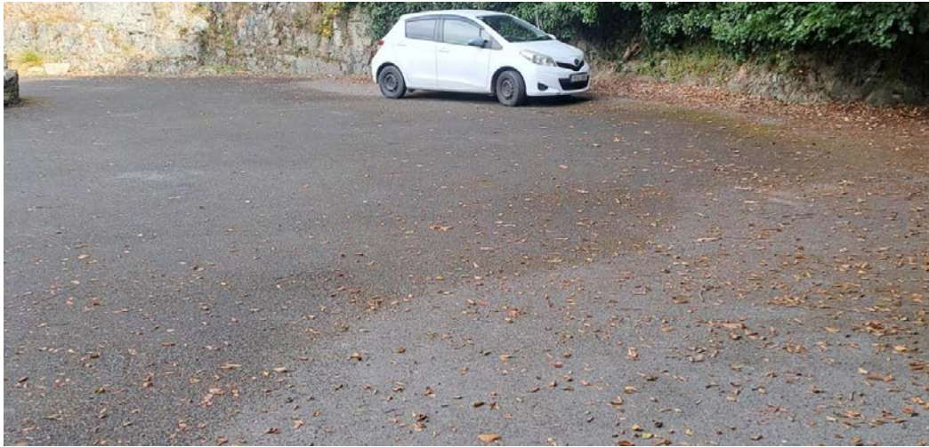
Apx Figure 28: Parking Area Associated with the Gort Scith Picnic Area
