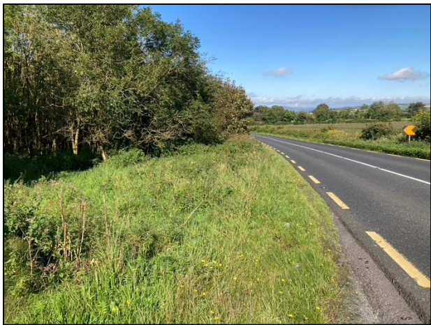
Figure 11: PDCZ 3A.1 looking north (above) and below looking south on N14
