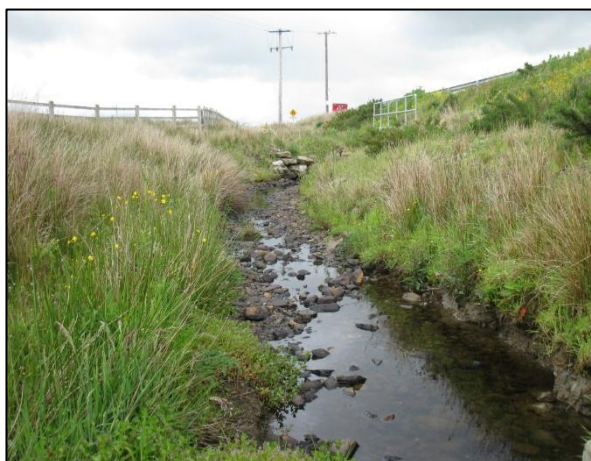
W1-02 (June 2020) Tributary of Burn Daurnett following N15 culvert upgrade.
