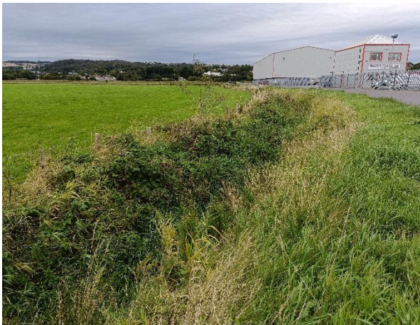
W2-16 (Sept. 2024) Milk Isle drain: virtually dry, vegetated, low-gradient drain.
