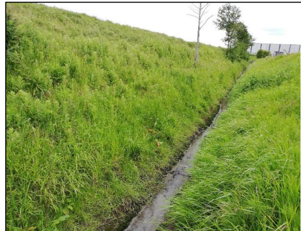
W2-22 (June 2020 and Sept. 2024) Typical embankment toe-drain at Bunnagee.
