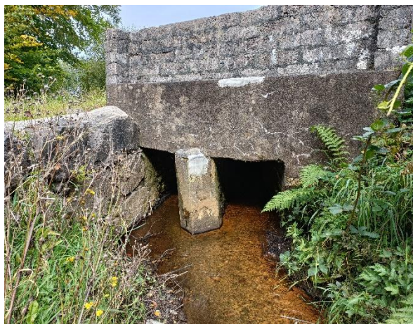
W1-11 (Sept. 2024) Magheracorran, view downstream at N13 culvert entrance. Trout observed.
