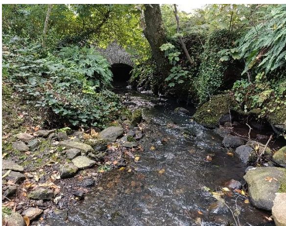
W1-20 (Sept 2024) Mullaghagarry, view downstream towards existing N15 culvert
