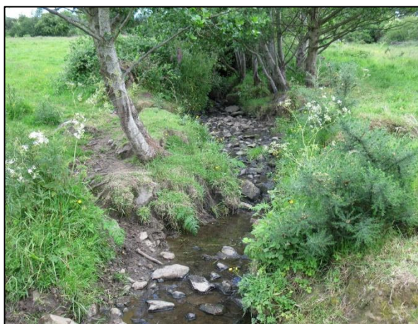
W2-04 (June 2020) Unnamed tributary of Swilly in Drumany - flows into screened pipe/culvert under existing road just downstream
