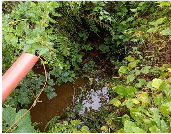
W2-09 (Sept. 2024) Stagnant outfall area from piped watercourse.
