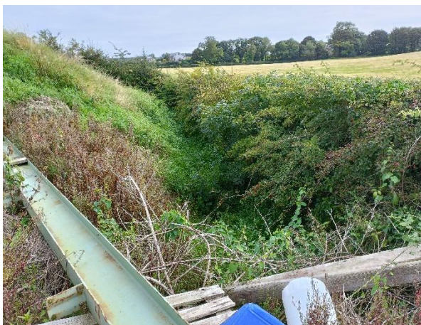
W2-23 (Sept 2024) Dromore 39, dry at crossing point, piped under industrial area access.
