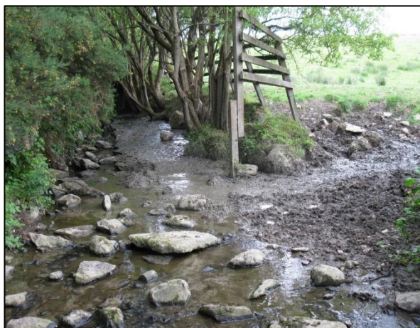
W2-12 (Sept. 2024) Farsetmore, downstream of existing N14 crossing showing polluted cattle access reach.
