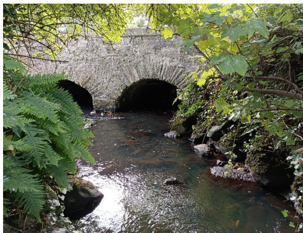
W1-20 (Sept 2024) Mullaghagarry, existing N15 stone arch culvert. Salmonids observed.
