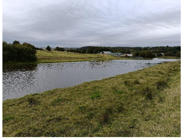
W2-18 (Sept. 2024) River Swilly crossing location, view downstream at high tide showing set back embankment area in foreground.
