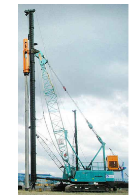
MOBILE PILING RIG
