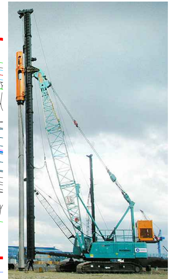
MOBILE PILING RIG
