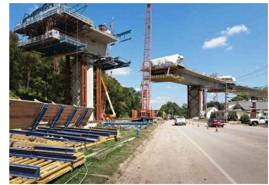
BALANCED CANTILEVER
